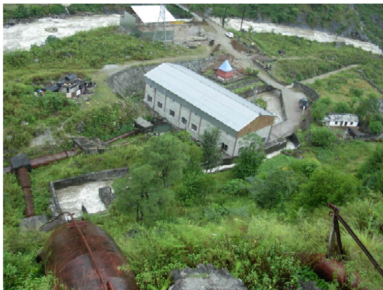
Fig.: 4.4: Spilling type surge tank and penstock system (Source: Alternate Hydro Energy Centre)
